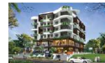
KINGDOM TOWER Thokkottu, Mangalore
