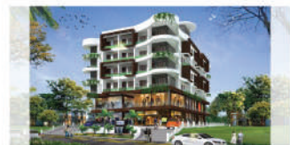
KINGDOM TOWER Thokkottu, Mangalore
